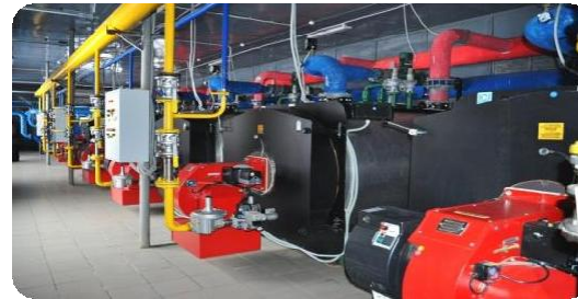
Boiler room modernization
