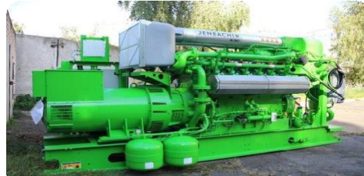
Cogeneration unit installation
